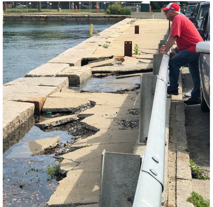
Broken concrete shows how badly repairs are needed at Storer Park Causeway and Pier.
