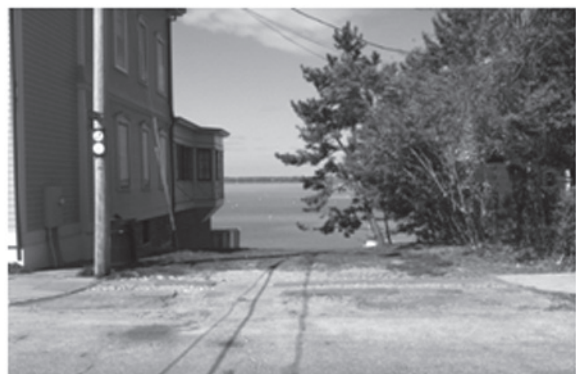
CHESTNUT STREET DRIFTWAY at Washington Street MATERIALS AND DIMENSIONS: Crosswalk: Bluestone and cobble Drift way: dirt and grass COMMENTS: This driftway has two strips of bluestone and two strips of cobble.
