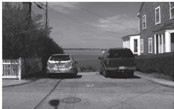
CHERRY STREET DRIFTWAY at Washington Street MATERIALS AND DIMENSIONS: Crosswalk: Bluestone evidenced at surface. Driftway: Asphalt roadbed leads to shoreline via concrete steps. COMMENTS: This driftway has bluestone and asphalt may be covering other materials at the crosswalk. The concrete steps at this driftway are incorporated into a concrete bulkhead.
