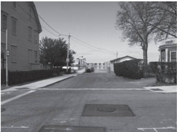
ELM STREET DRIFTWAY at Washington Street MATERIALS AND DIMENSIONS: Crosswalk: Bluestone and cobble set in concrete Driftway: asphalt to shoreline COMMENTS: This driftway has two strips of bluestone and one strip of cobble set in concrete.
