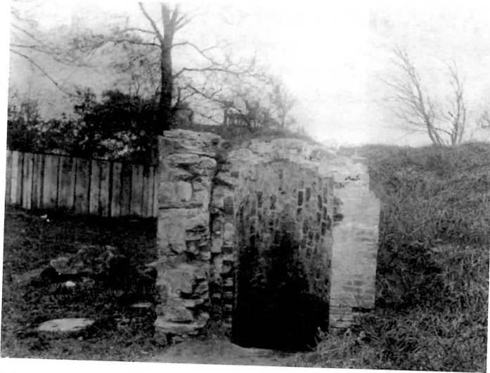
Figure 4 — Entrance to dungeon at Fort Greene — looking south
