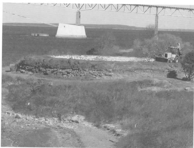
A backhoe was purchased to remove the cement supporting the roof and the earth that covered the exterior stone wall. March 2006
