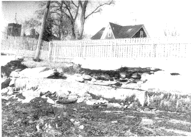
The seawall at Hunter House
